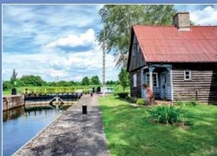
Śluza Lipica Schleuse in Lipica
